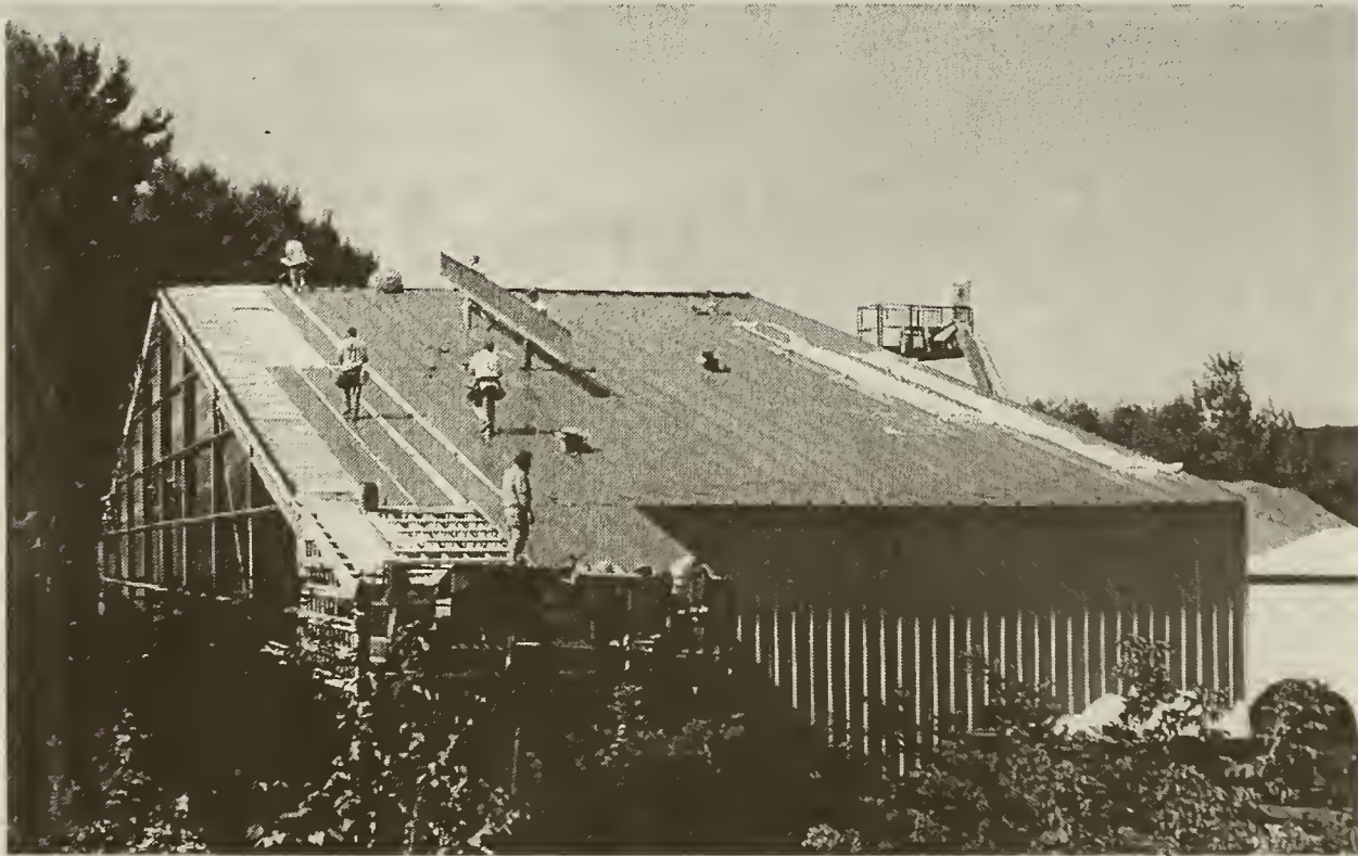
September 13, 2004. Installing the roof by Riess Construction of Plymouth, NH.
